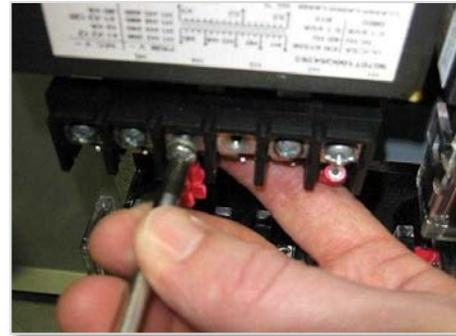
7. Install the extra screw back onto the old PT location and tighten.
