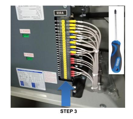
NOTE: Please note wire locations before disconnecting for proper re-installation.
