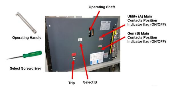
Once both Utility and Generator supplies are de-energized the following procedure can be used to operate the Transfer Switch Manually.
