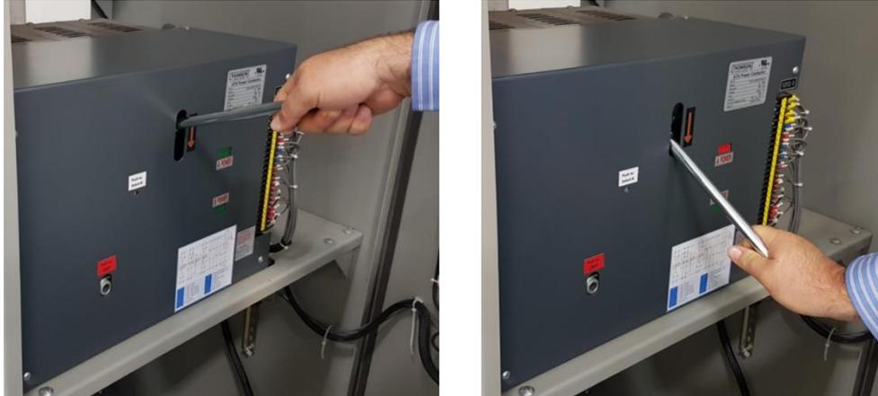
5. Once ATS is manually operated to the Utility “ON” position, remove the operating handle from the Power Contactor and secure them away from any live power sources.
