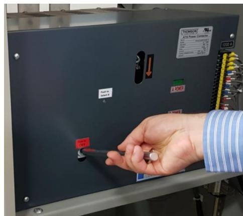
4. **Close Utility (Side A) Main Contacts** by inserting the operating handle onto the Power Contactor Operating Shaft and move in the direction shown below until the Utility Main Contacts latch closed as shown by the Utility “ON” indicator.
