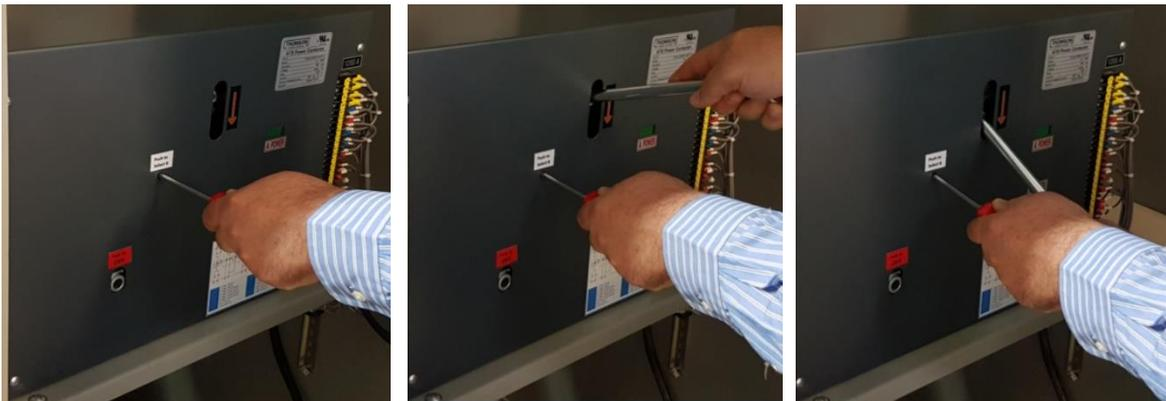
5. Once ATS is manually operated to the Generator "ON" position, remove the operating handle & screwdriver from the Power Contactor and secure them away from any live power sources.
