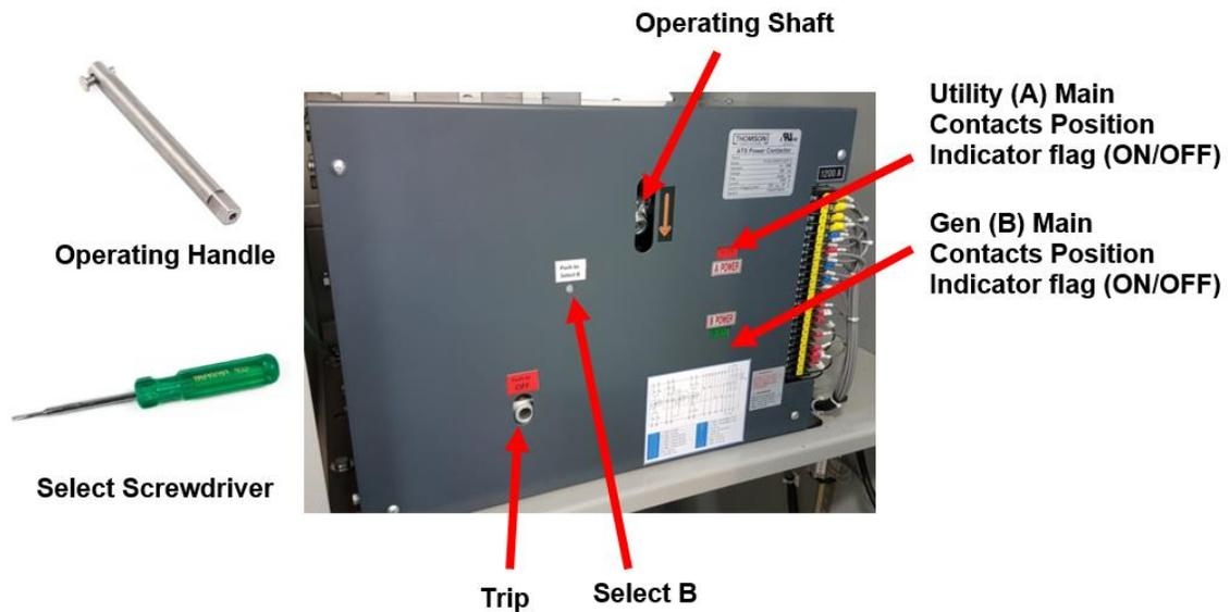
Once both Utility and Generator supplies are de-energized the following procedure can be used to operate the Transfer Switch Manually.
