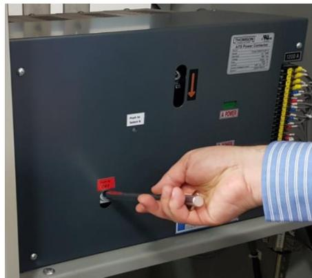
4. **Close Generator (Side B) Main Contacts** by using both operating handle and screwdriver simultaneously as described below:
